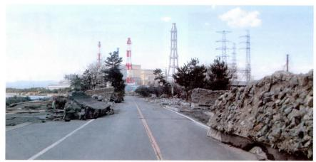
Breakwaters were swept over the street by the tsunami in Iwama district. Chimney shown in the photo is from the Nakoso Power Plant, Joban Joint Power Co., Ltd. The power plant was also damaged by the tsunami, but restored their main generators 8 & 9, and then they also recovered the generators 6 & 7 which were stopped, and supplied electricity to TEPCO and Tohoku Electric Power Co. 25<sup>th</sup> March Photo courtesy: Ms. Akemi Itoi
