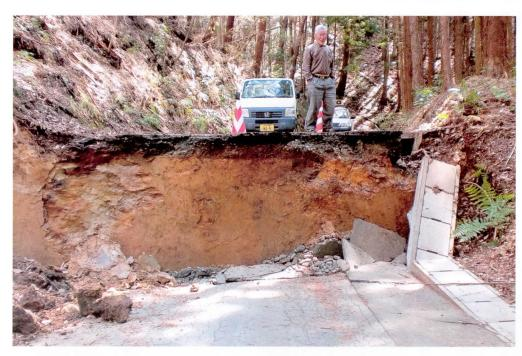
There are multiple faults running through underground Tabito machi. The April aftershocks created a level difference of 2 metres in many places.
