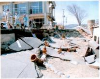
Tsunami sank the roads and made the buried water pipes visible Kageisobashi, Hisanohama (14<sup>th</sup> April)
